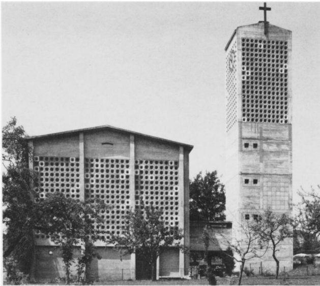
Fig. 5. Egon Eiermann, Matthäuskirche, Pforzheim, 1952–1956, Exterior, altar side (Artur Pfau, Mannheim; The Architectural Collection of the University of Karlsruhe).
