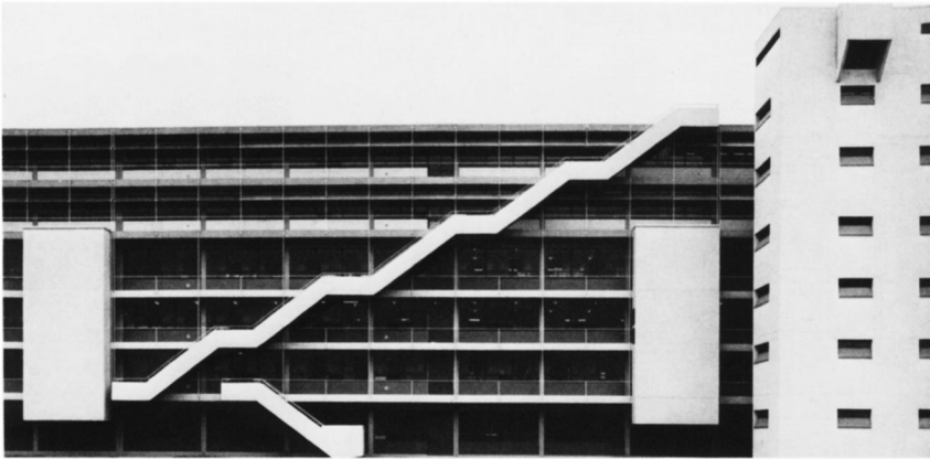
Fig. 40. Egon Eiermann, Mail Order Warehouse for the Josef Neckermann KG, Frankfurt am Main, 1958–1961 (Horstheinz Neuendorff, Baden-Baden; The Architectural Collection of the University of Karlsruhe).
